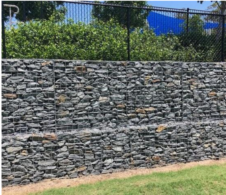
Fig 57. Illustrative example of the use of stone filled gabion baskets to act as an architectural solution for an acoustic barrier
